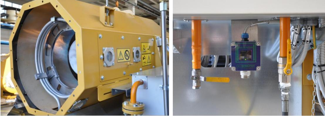
Figure 4 – On the left: detail of operation of the air vein burner - on the right: detail of the shut-off valves and electronic gas leak analyser.
